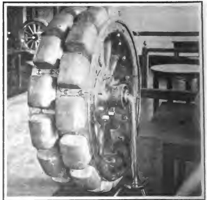
Kelly-Springfield Sectional Rubber Tire for Heavy Duty
